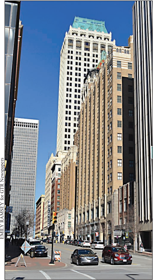
BOSTON AVENUE: A north view of Boston Avenue in downtown Tulsa's Deco District. Downtown Tulsa boasts some of the most renowned art deco architecture in the country.
