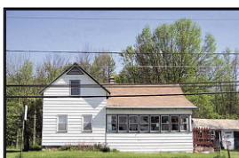
Cicero $439,000 Commercial use, 2.95 acres located in high traffic area among other successful businesses. Sandra L. Farrands 315-952-8216 (C)
