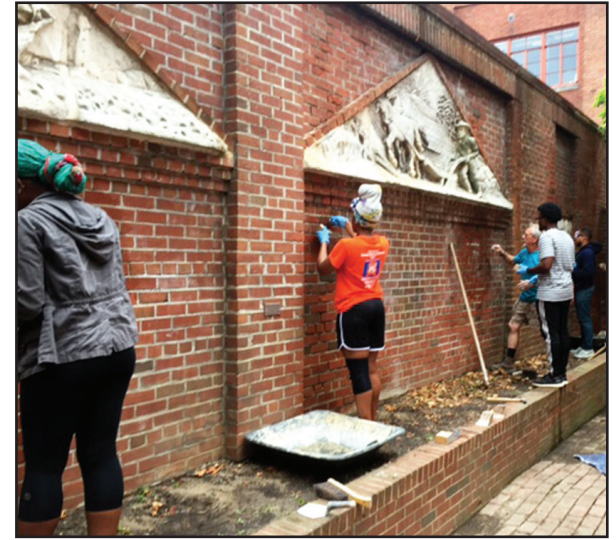
Students repointing the brick wall
