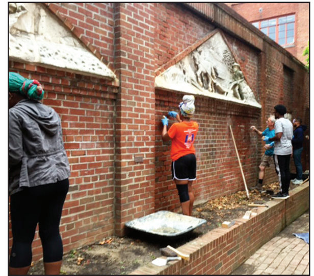
Students repointing the brick wall
