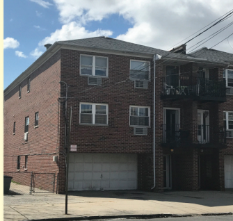
PELHAM BAY LARGE 4 FAM + FULL BSMT 3 ONE BED ONE BATH APTS & 1 THREE BED TWO BATH APT 2 CAR GARAGE CORNER LOT 4 HEATING SYSTEMS $1,050,000
