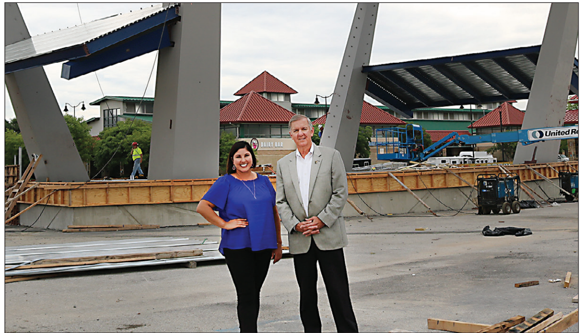
OVERSEEING PROGRESS: Present at the construction at the Tulsa State Fair are Amanda Blair, Tulsa State Fair manager and Expo Square COO, and Mark Andrus, president and CEO of Expo Square. In the background is construction for the greatly expanded Oklahoma Stage. Other improvements include the new Mega Barn, Pavilion exterior updates and improvements to the Tulsa State Fair entrance gates.
