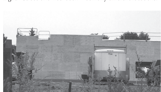
Northwoods Crossing in under construction in Baxter.
