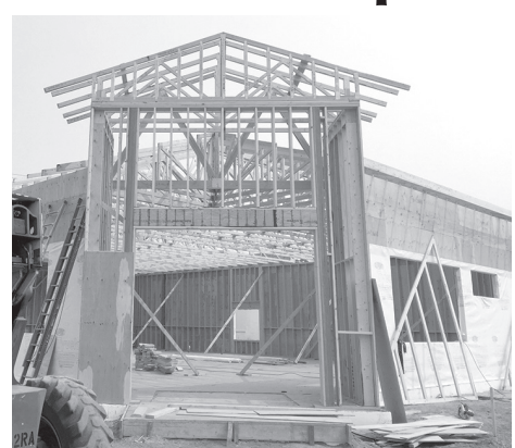
Thrifty White Drug in Brainerd is under construction.
