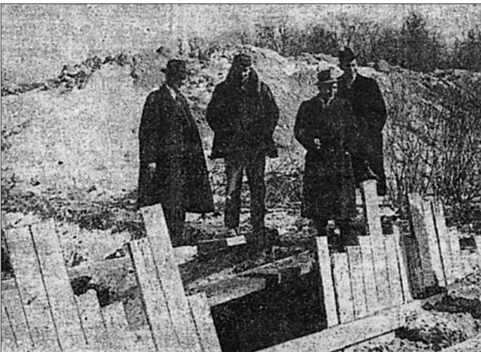
Left to right are C. E. Broughton, founder of the Marsh Park, Harold Meinen, superintendent of construction, Dick Jarvis, sports editor of The Press and M. R. Ellis, reporter inspecting one of the by-passes that had been used to carry off water from the marsh to ease the pressure on the original dam while the new dam was constructed.
