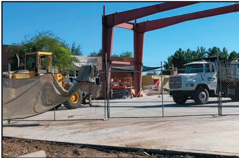
The bulldozers and heavy equipment have left a Tempe church after workers dismantled a longstanding steel frame from an abandoned construction project. — Wrangler News photo
