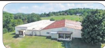
#873 - Building has two sides. Larger side is approximately 20,000 sq ft. with 19'4" peak and 12' on sides and has sprinkler system. The smaller side has approximately 7500 sq ft with 15' height and 7500 sq ft with 11'3" height. Each side has dock doors. MLS#1666214 $175,000
