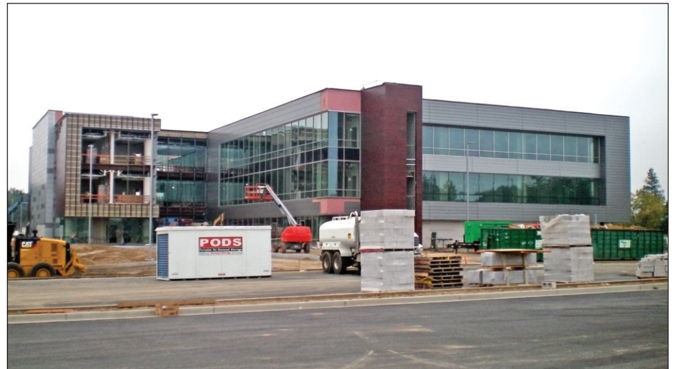
The new Veteran's Clinic, shown here under construction at Silver Creek Valley Place, will replace the old clinic located at 80 Great Oaks Blvd. in south San Jose.
