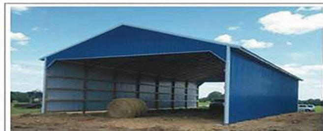
40x84x14 steel trusses, 2x6 purlins and girts, 6x6 pressure treated posts, #1 29 ga. painted walls and #1 29 ga. galvalume roof.
