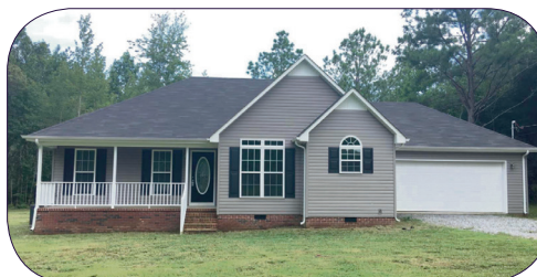
42 Hattie Dr. - Beautiful home and 5.05 acs. features large Lr w/ double trey, M. B/R has double trey and walk-in-closet, 3 B/Rs, 2 full baths, large kitchen with island, 2 pantries, all appliances, vaulted ceiling, attached garage, fenced back yard, storage building and privacy. Convenient to Huntsville. MLS#1993636 $168,900
