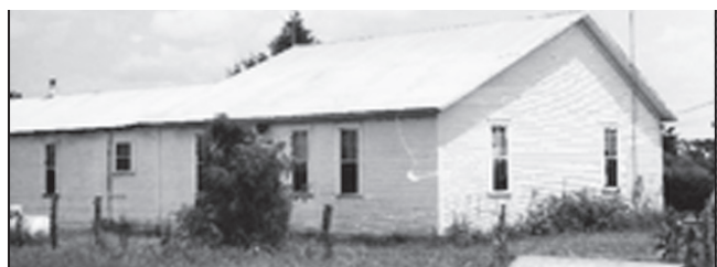
Old farm house at Porter Farm House
