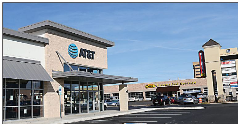
READY FOR BUSINESS: The rebuilt AT&T store has officially opened for business in the Highland Shopping area. The address is 5505 E. 41st St.
