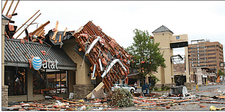
TULSA TWISTER: The 2017 Tulsa tornado took place on Aug. 6. Major damage was inflicted on the Highland shopping and office area in southeast Tulsa.
