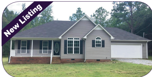
42 Hattie Dr. - Beautiful home and 5.05 acs. features large Lr w/ double trey. M. B/R has double trey and walk-in-closet, 3 B/R's, 2 full baths, large kitchen with island, 2 pantries, all appliances, vaulted ceiling, attached garage, fenced back yard, storage building and privacy. Convenient to Huntsville. MLS#1993636 $168,900
