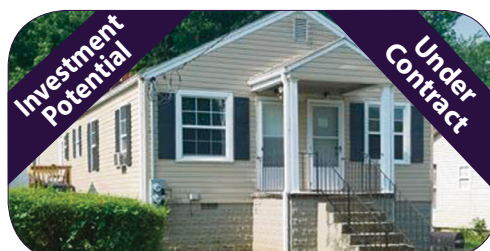
1006 College St. W. - This duplex is located just off the town square. This property is close to shopping, restaurants and local schools! This property has a history of a good rate of return for investors. This property would make a wonderful investment for 1st-time flippers or someone looking to get into the rental house market. New paint and carpet! MLS#1935398 $65,000
