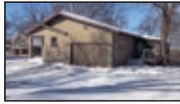
415 E. Oak St ~ Redwood Falls River Valley view! $199,000
