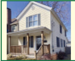
423 3rd St. Fairport Harbor $107,400
