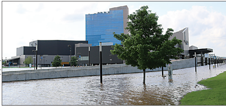
HIGH WATER ALONG RIVERSIDE: Arkansas River water threatened River Spirit Casino Resort in Tulsa, but the resort withstood serious damage. River Spirit CEO Pat Crofts reported, "While the photos and videos may appear alarming, we want to reassure the public that River Spirit, including the 27-story hotel, Margaritaville and Ruth's Chris restaurants, and both our gaming floors remain unaffected by the water surrounding our property." He added, "River Spirit and all of our facilities are structurally sound. The design and engineering of River Spirit was built to withstand a 100-year flood and any severe weather-related event."
