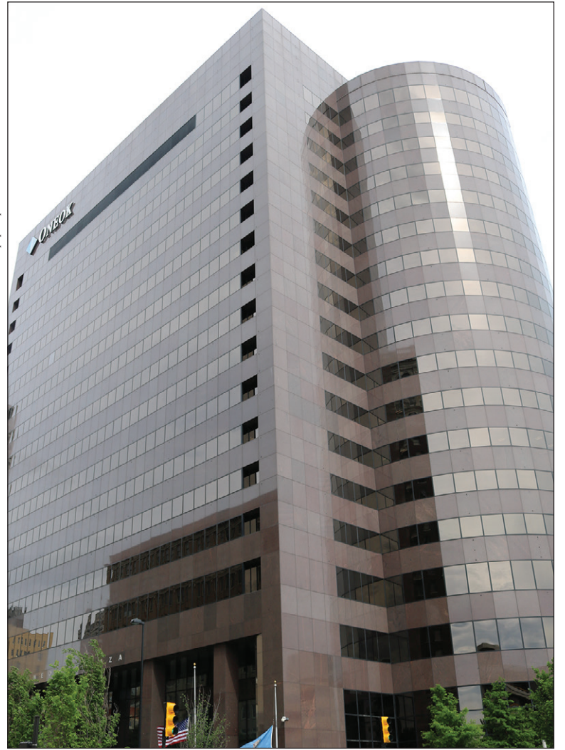
GREAT ASSET: The Oneok Plaza tower is a 17-story building occupying the north half of the block running from South Cheyenne and South Boulder avenues and West Fifth and West Sixth streets.
