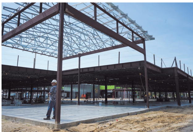
Showell School under construction. Photo by Worcester County Schools
