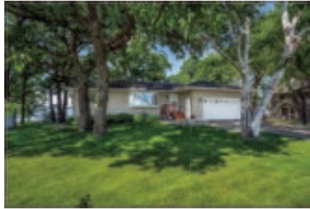
Norway Lake | 3956 189th Ave NW, New London $369,000 | MLS# 5200631 3 bedrooms, 2 bathroom / 100 ft of shoreline
