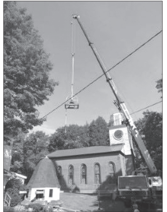
The dome that replaced the tower in 1916 was removed in 2012. Plans are underway to replace the original tower.
