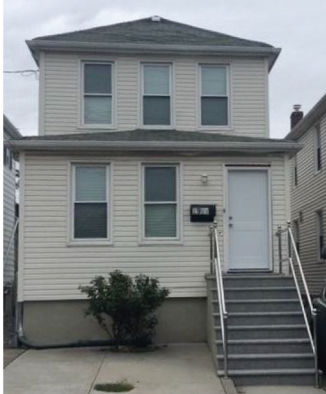
Throgs Neck -1 Family Detached Frame, 6 Rm, 3 Bdrs, New Kitchen w/ Stainless Steel Appliances, New Baths, Ceramic Tile, Oak floors, Finished Basement w/ one Full bath, Driveway. $579,000
