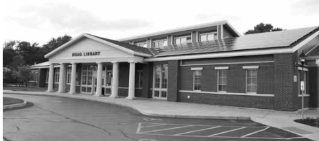
The Hoag Library opened in July 2012 on South Main Street in Albion.
