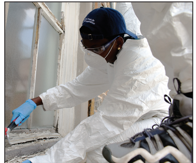
Zahaira Williams works on restoring a window at MSU’s Memorial Chapel
