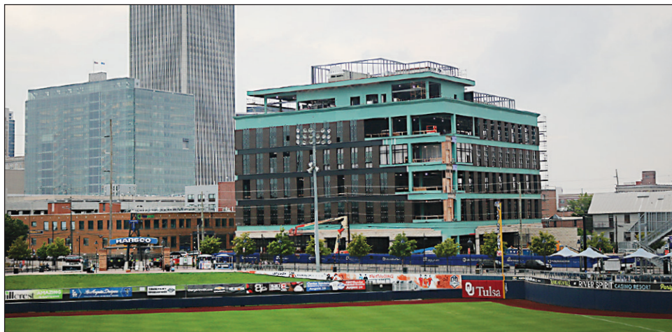
GOING UP: The new Vast Bank headquarters building across from ONEOK Field in downtown Tulsa is taking shape. Expected to open in December, the building will include a rooftop “In the Raw” sushi bar, rotating art installments and office space.
