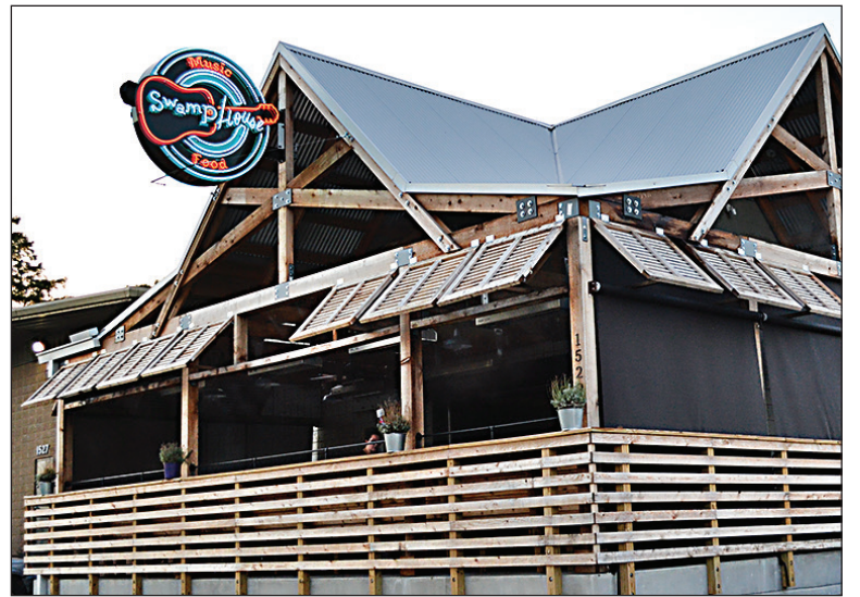
STUDIO ROW LOCATION: SwampHouse, 1529 E. 3rd St., opened in May in one of Tulsa's up-and-coming neighborhoods, located near 3rd Street and Trenton Avenue.
