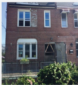
1808 PATTERSON AVE LAND & 2 FAMILY REHAB $799K
