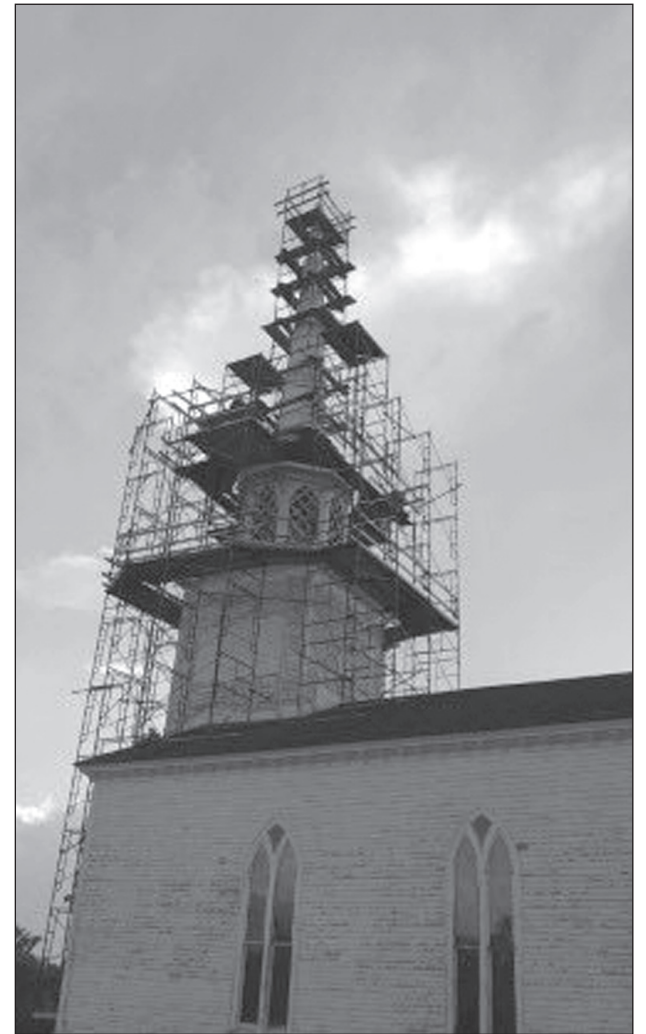
Meeting House with scaffolding
