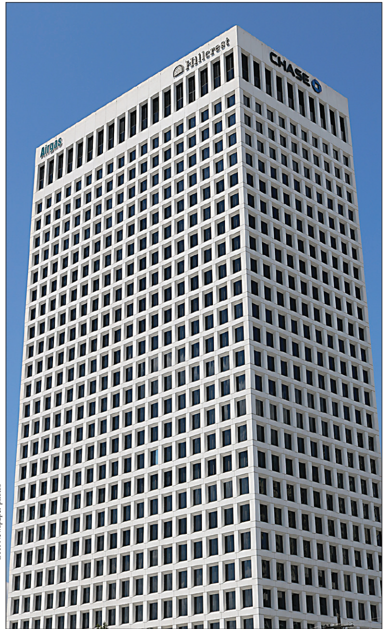
STATELY LANDMARK: The Robinson Park Building stands at 28 stories with a geometric façade that is achieved by a waffle-like grid of deeply recessed glass openings.
