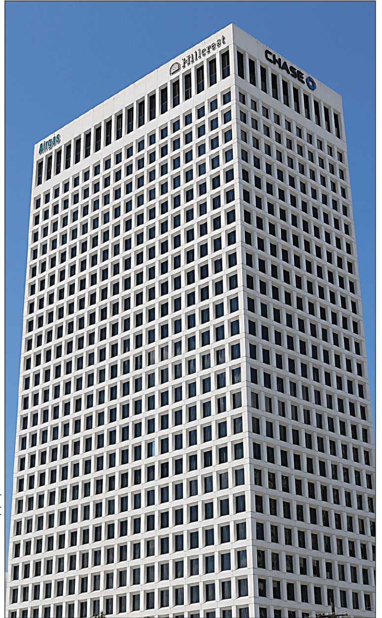
STATELY LANDMARK: The Robinson Park Building stands at 28 stories with a geometric façade that is achieved by a waffle-like grid of deeply recessed glass openings.
