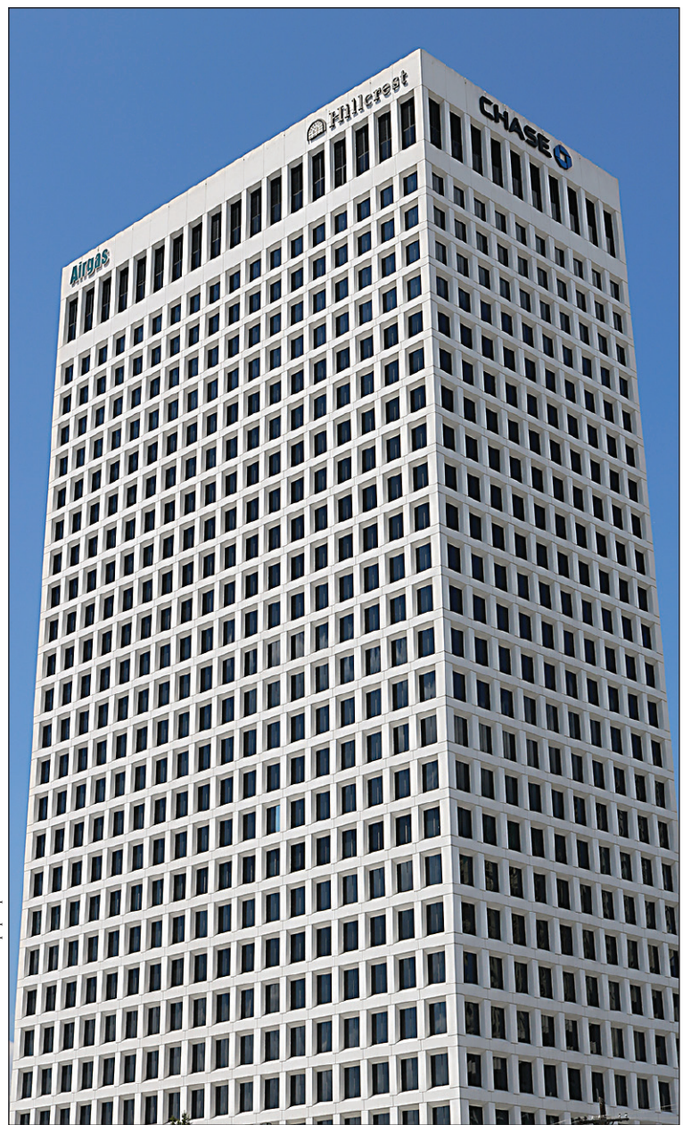
STATELY LANDMARK: The Robinson Park Building stands at 28 stories with a geometric façade that is achieved by a waffle-like grid of deeply recessed glass openings.
