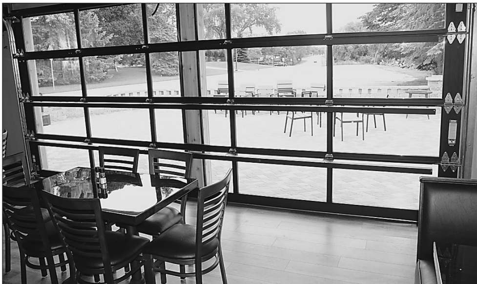
A new double wide glass overhead door constitutes the south wall of the dining room at Route 67 in Elkhart Lake. The door opens to a brick patio area. A fan system to the side of the door keeps insects from flying into the dining room when the door is open, as it has been several times in recent weeks. The view from the dining room and the patio looking south is of traffic on STH 67, which is fitting considering the name of the establishment. Pictured below, Head Chef Devon Dederling and Managing Partner Angela Girard have helped make huge changes to the Elkhart Lake restaurant/bar now known as Route 67.
