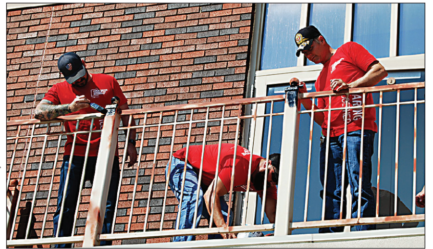
PAINTING THE RAILING: This four-person team of PSO volunteers was tasked with painting the railing on the second-floor balcony of the museum.
