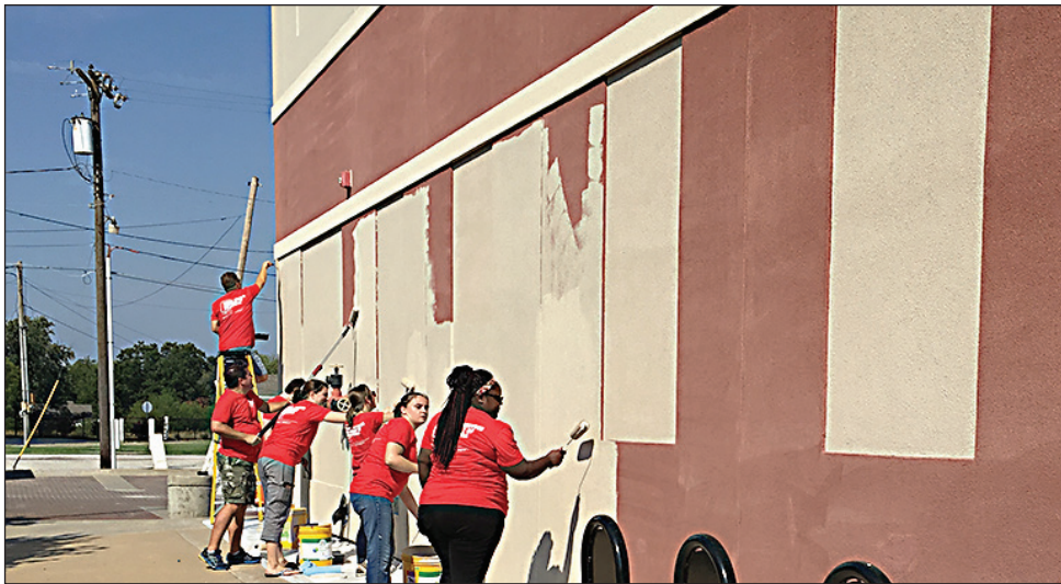
PREPPING FOR THE MURAL: This wide shot shows the south exterior wall of the museum where PSO employee-volunteers are prepping the wall for a mural that will be painted later.
