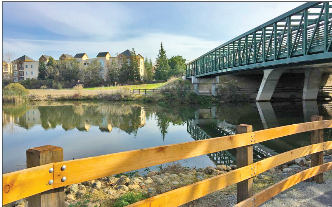
A 600-foot undercrossing at Coleman Road allows residents to walk all the way around Lake Almaden.
