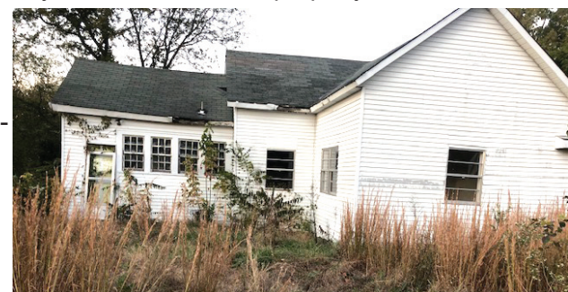
The council authorized the demolition of a house at 403 Waterloo Road.
