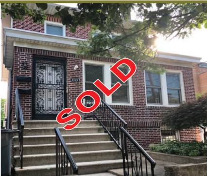
Throgs Neck - 2 Family - Detached Brick, 5 rooms/ 3 Bed, Over 5 Rooms / 2 Beds, Over 3 Room/ 1 Bed (Basement) 50 X 100 Lot, Hardwood Floors, New Anderson Windows. Great Investment Property. Individual Boiler / Water Heater. Ask for Gilda
