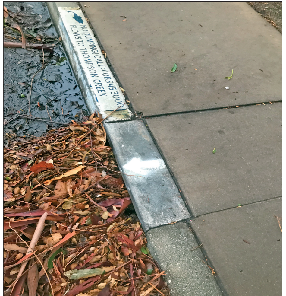
Debris clogged drain on Yerba Buena Road.
