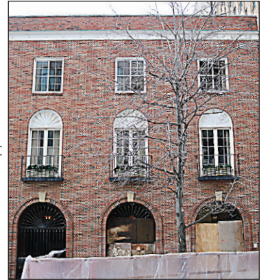
ARCHITECTURAL RENEWAL: The University Club Building is located at 114 E. 5th St. in Tulsa directly across the street from the newly remodeled Tulsa Club Hotel. The University Club Building is currently experiencing its second remodel.
