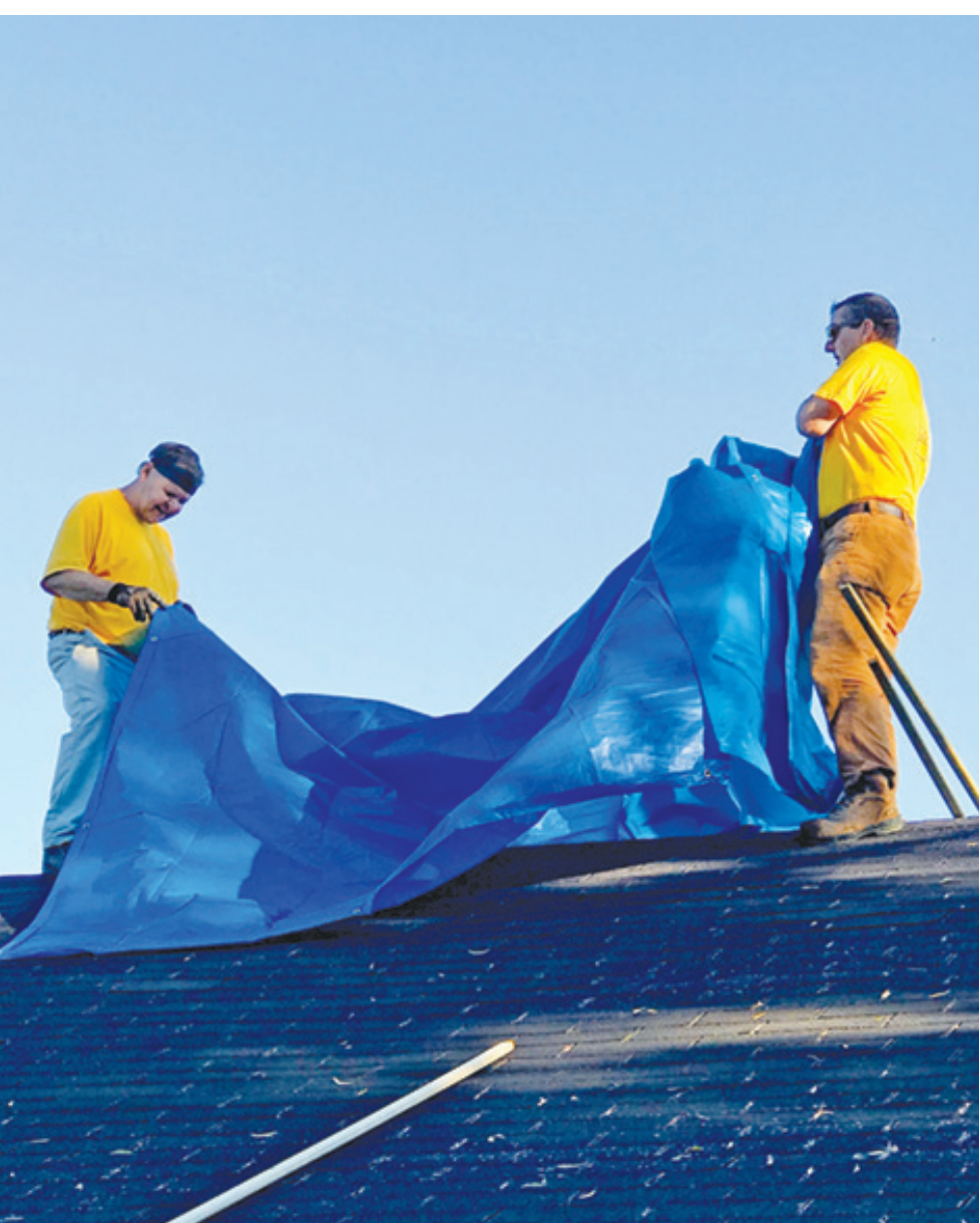
Disaster Relief Team members are shown tarping a roof in Texas.
