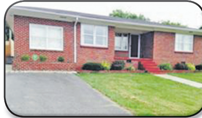
1604 Washington St. W. - Check out this great starter or retirement home in the city limits of Fayetteville. Could be commercial business if desired. Nice 3 bdrm, 2 bath brick home, beautiful knotty pine walls, CHA, lots of updates, new wooden privacy backyard fence, paved drive. MLS# 1553353 $92,000 CATHY WORRILOW 931-374-5050
