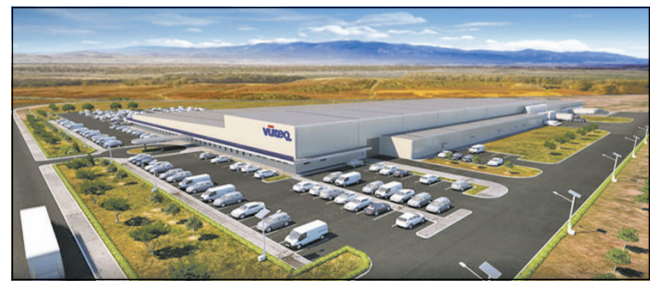
An artist's rendition of the planned Vuteq USA plant under construction off Greenbrier Parkway in Huntsville-annexed Limestone County. The 200-employee plant will produce interior and exterior plastic-injected parts and sub-assemblies for Mazda Toyota Manufacturing USA. [COURTESY ILLUSTRATION]
