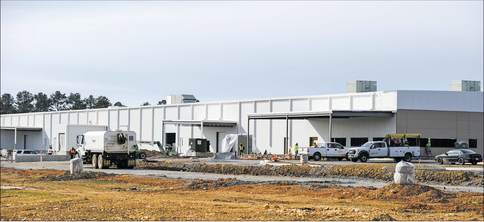
Construction of the Toyota Boshoku plant in Athens continues in late January. [JERONIMO NISA/DECATUR DAILY]
