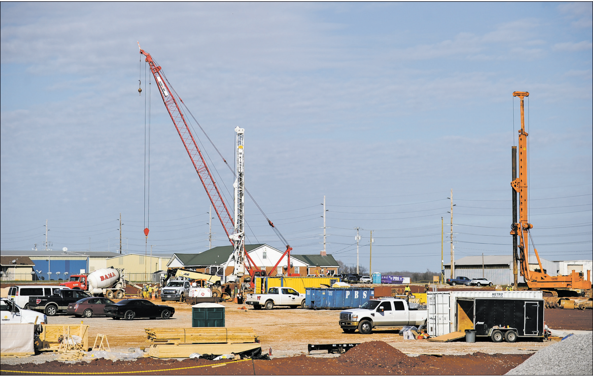
Construction continues on the Vuteq USA plant on Greenbrier Parkway in Limestone County. The plant eventually will have 200 workers. [JERONIMO NISA/DECATUR DAILY]
