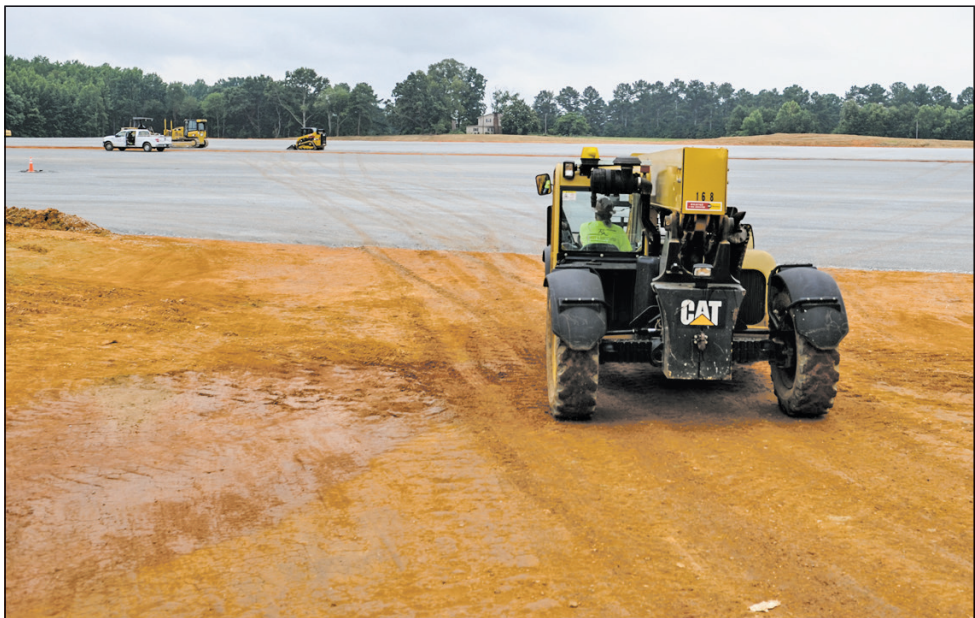
Workers make progress in June at the new Toyota Boshoku America plant's construction site in Athens. [JERONIMO NISA/DECATUR DAILY]
