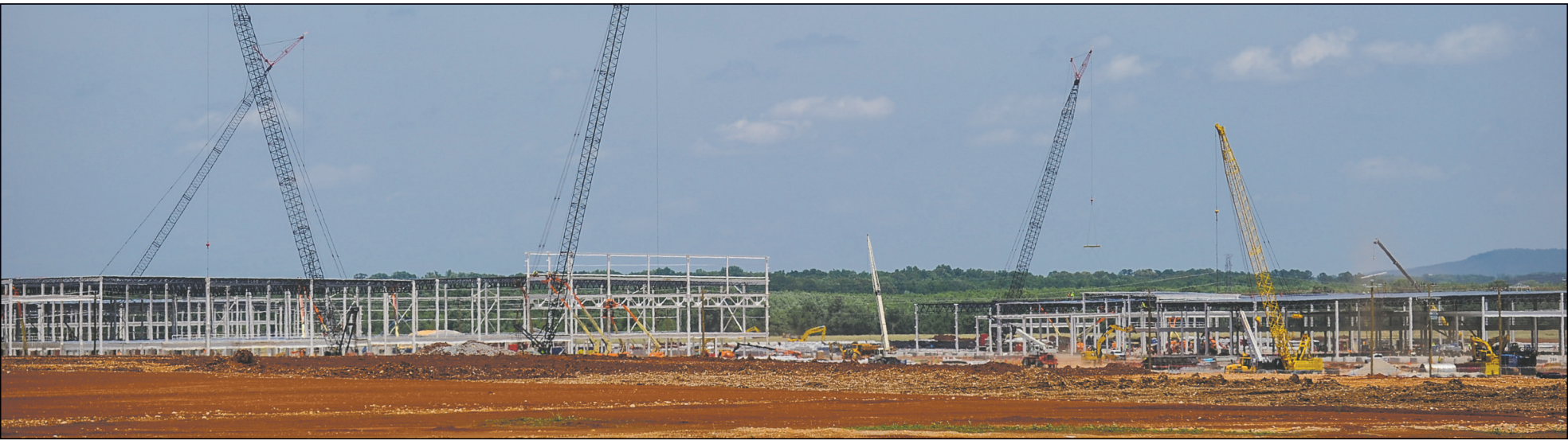
Cranes were numerous at the Mazda Toyota Manufacturing USA construction site in May. The DNUS plant will be situated on the Mazda Toyota site for quick delivery. [JERONIMO NISA/DECATUR DAILY]
