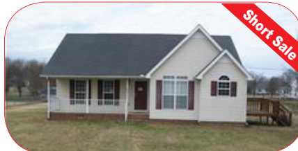
93 McAlister Rd. - "2004" home in Highland Rim school district...3 BRs, 2 BAs. Large kitchen w/vaulted ceiling. Large family room. Deck and covered front porch on 1/2 ac. lot. MLS#1603250 $76,000
