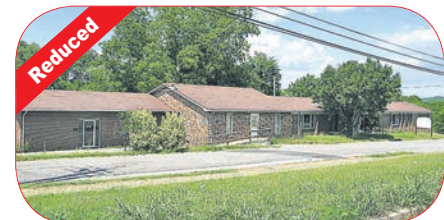
615 Maple St. W. - Approx. 4,812 sq. ft. building with kitchen and bathrooms. 2 Lots on .85 ac. Paved parking. MLS# 1539043 $59,000
