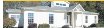
T-102: 1521 Ardmore Hwy 110, Taft. Situated on 7.1 acres, this updated home boasts 2460 SF, 4 BR/2 BA, open floor plan, 18' ceiling in LR, recessed lighting, laminate flooring, office/den w/ wood-burning stove, master w/ wood-burning FP. 16x20 detached building w/ work stations in place. 28x26 concrete pad is poured for detached garage. $209,900.
