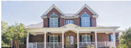
T-092: 983 Veto Rd, Prospect. Donald Gardner plan w/ numerous amenities, hardwood flooring, extensive trims & crown moldings, recessed lighting, granite counters, custom cabinets w/ raised panel doors, Andersen windows, Rinnai water heater, smooth ceilings, gas log FP, Jenn Air SS appliances, security system, partially finished basement w/ rec room, attached garages. 3724 SF, 4 BR/4.5 BA. 9.2 Acres. $559,000.
