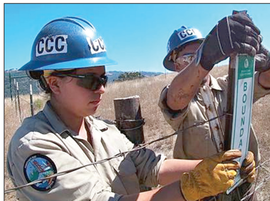
Above left: CCC Monterey Bay Corpsmembers Amanda Romo and Julian Burgos install a boundary marker along the perimeter fence of the new Coyote Canyon Park, after removing barbed wire and t-posts from a hillside in Coyote Canyon.
