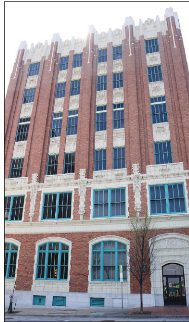
GOTHIC ENTRANCE: The 424 S. Detroit Ave. entrance featured the Gothic style of the time.
